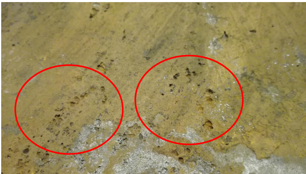
Figuur 5-3: putcorrosie dieseltank Oldebroek
